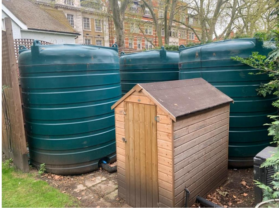
Existing Irrigation Tanks and Pump House in Groundkeepers Lodge garden
